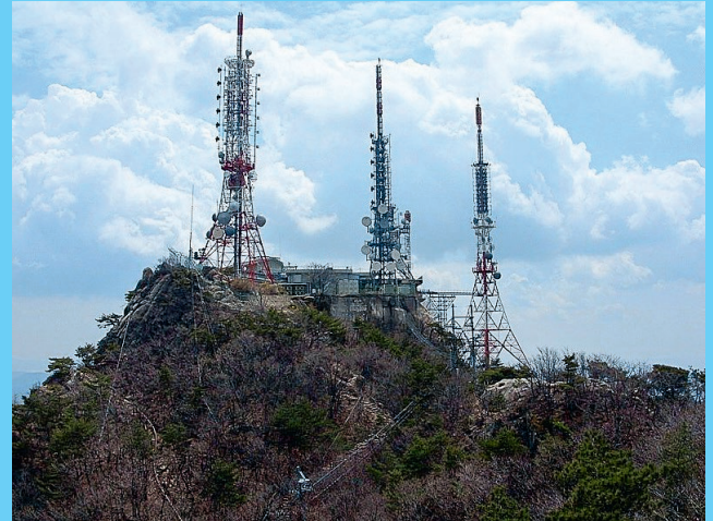
The KBS antenna tower (left) is used to broadcast the world's first terrestrial 4K programs.
