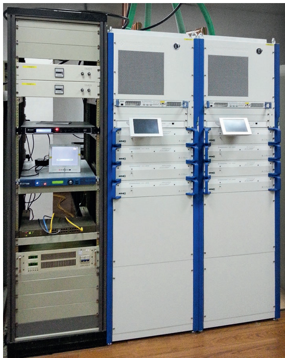
Two of the R&S®THU9 liquid-cooled high-power TV transmitters that provide the southern Chinese province of Hunan with digital television.
