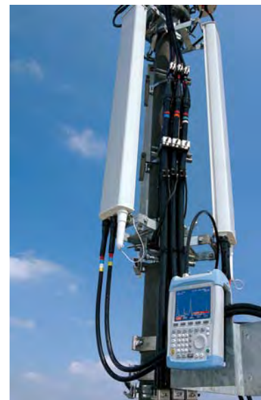
FIG 8 The R&S®FSH3, the do-it-all solution for measurements required during installation and on-site maintenance, used for measuring a mobile radio antenna.
